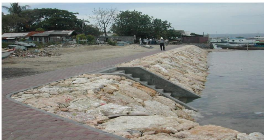
Gambar 8. Penguatan Lereng ( Revetment )
